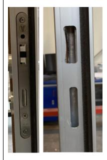
Detailed views of lock in active leaf (left) and strike plate in inactive leaf (right)
