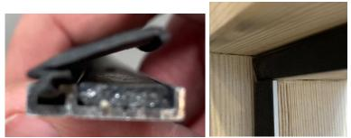
Detailed views of frame seal cross section (left) and mounting position (right)
