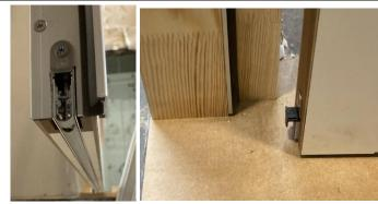
Detailed views of drop down seal (left) and actuation (right)
