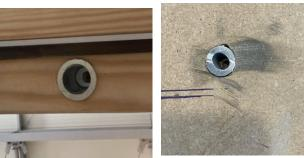
Detailed views of strike plates for top (left) and bottom locking (right) of inactive leaf
