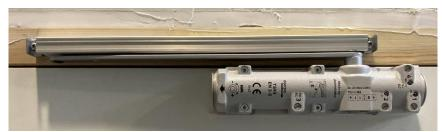
Detailed view of door closer with sliding rail
